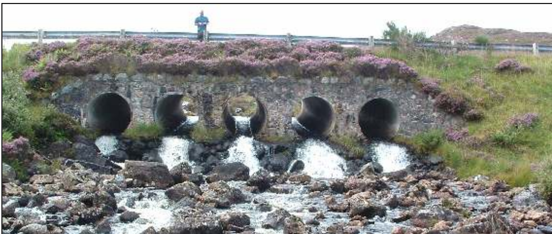
One of few man-made obstructions to fish passage in Wester Ross: the culvert beneath the A832 on the Allt Bad an Luig near Second Coast (Gruinard Bay) is too steep and is impassable to sea trout.
